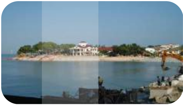
Reclamation works are approaching completion with protective rockbound in place.
