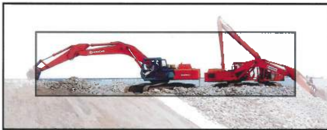
construction in progress : March 2004
